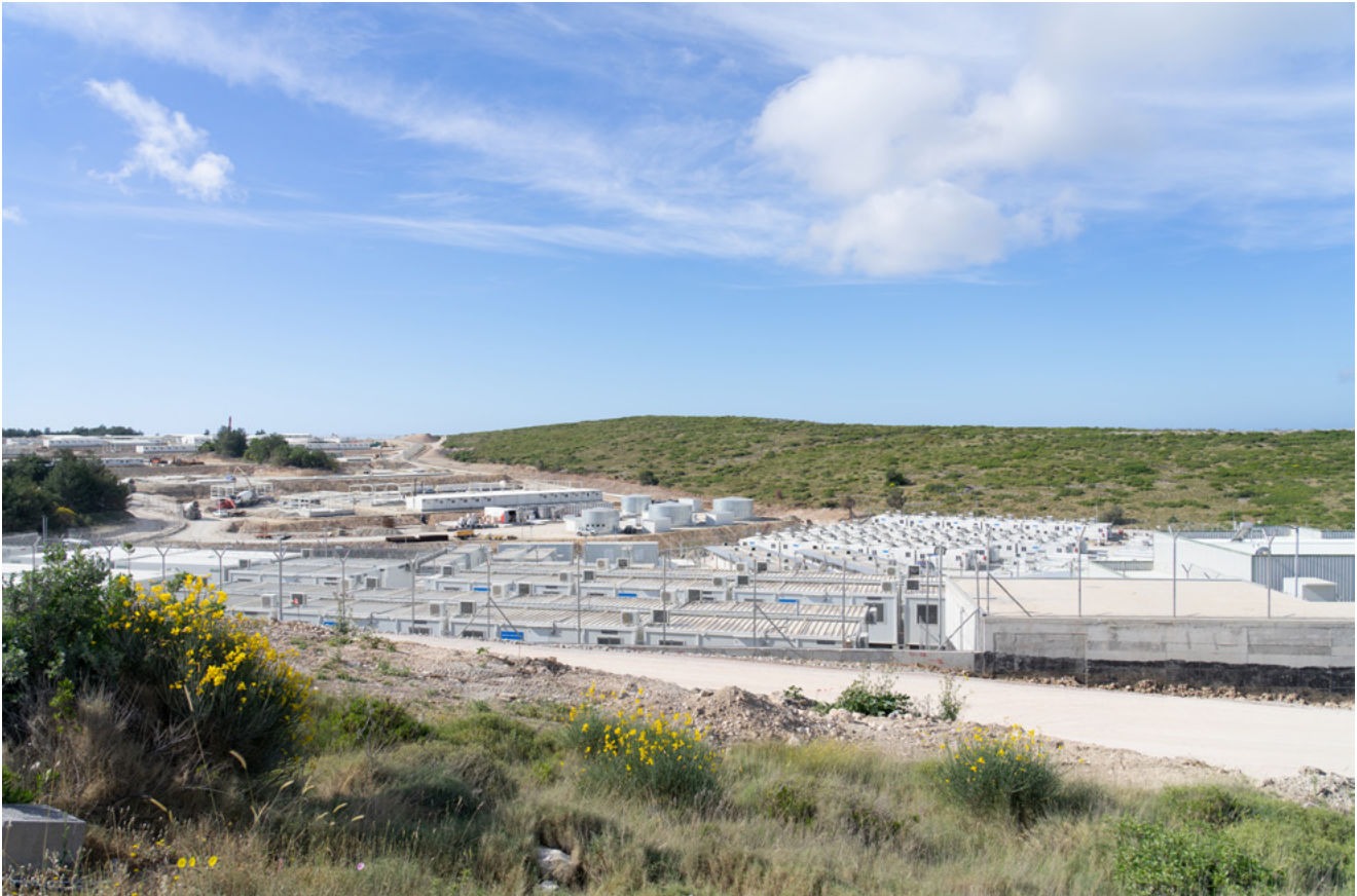
A view of the new Multi-Purpose Reception and Identification Centre, Samos, May 2021, © DORA VANGI/MSF
